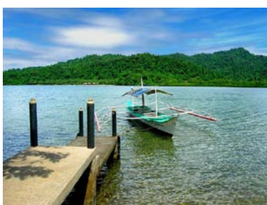
View of concrete boat pier
